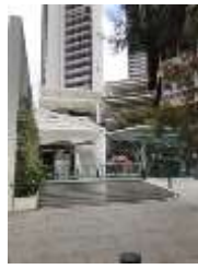
The entrances of Ege Perla buildings (Source: Zeynep Soysal's Archive, May 2019)
